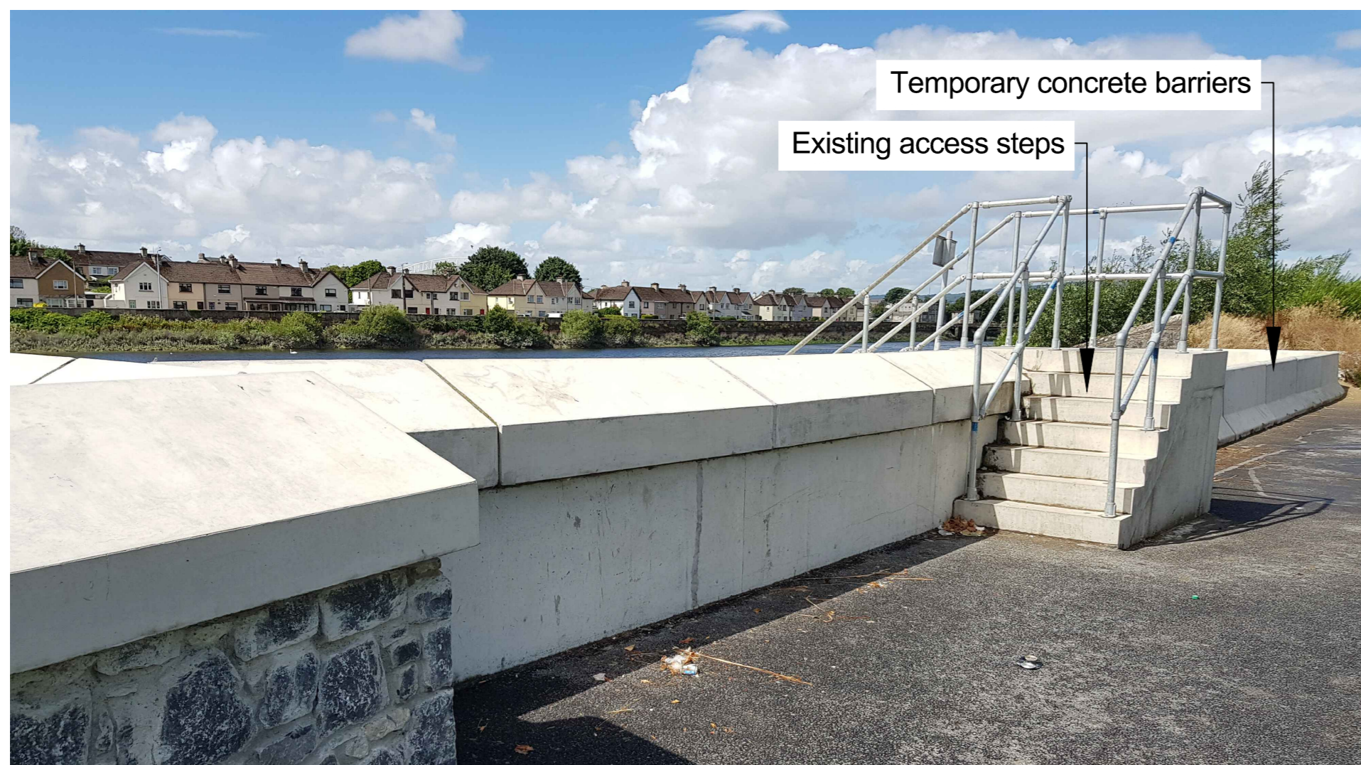
Existing concrete walling and barriers at Verdant Place Steps (KIFRS-A-001)
